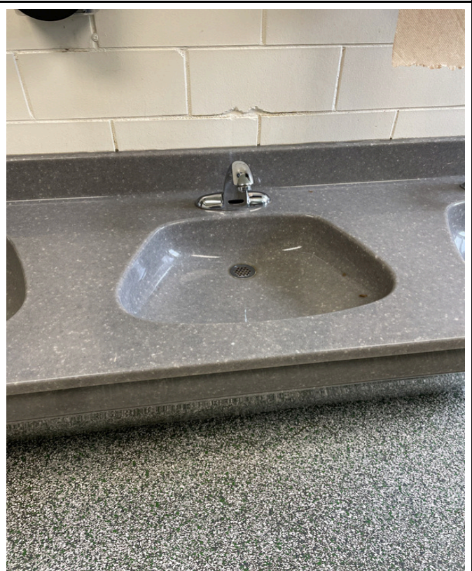
5/8/2024 - 527-17 - High School - Main Hallway Men's Restroom Center
