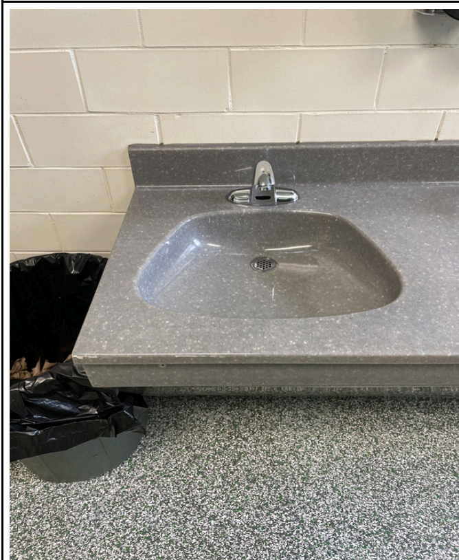
5/8/2024 - 527-16 - High School - Main Hallway Men's Restroom Left
