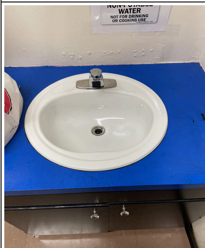
5/8/2024 - 527-5 - AG Building - Room F100b
