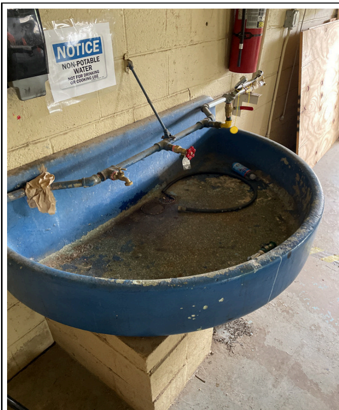
5/8/2024 - 527-1 - AG Building - Shop East Wall
