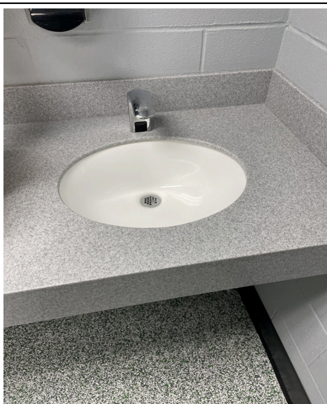
5/8/2024 - 527-6 - 5th/6th Grade - Men's Restroom Right
