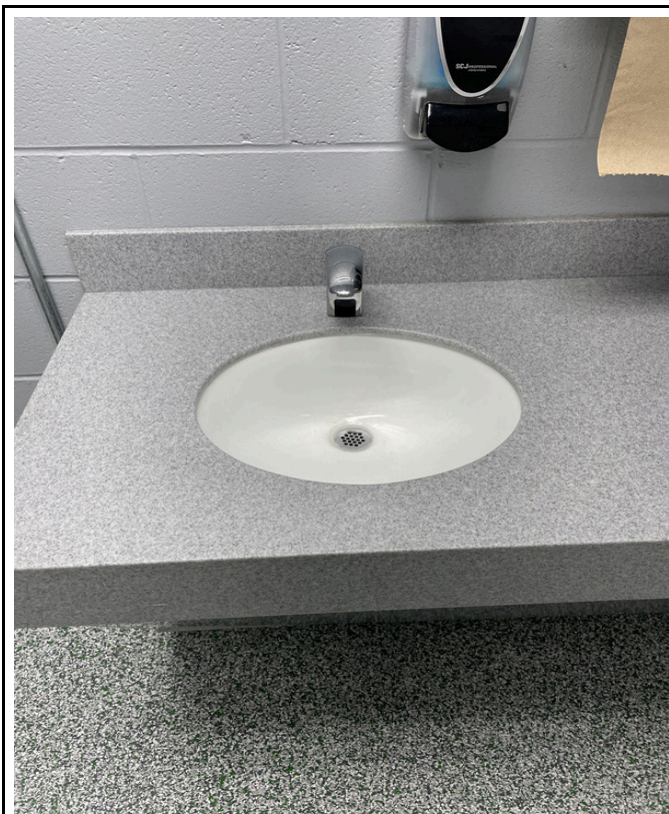
5/8/2024 - 527-5 - 5th/6th Grade - Men's Restroom Left
